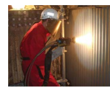
Protecting boiler tubes for the Power Generation Industry.
